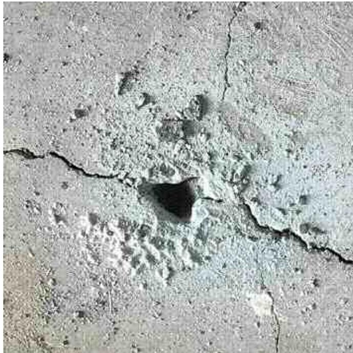
**Image 8** Drill Hole with radiating cracking
