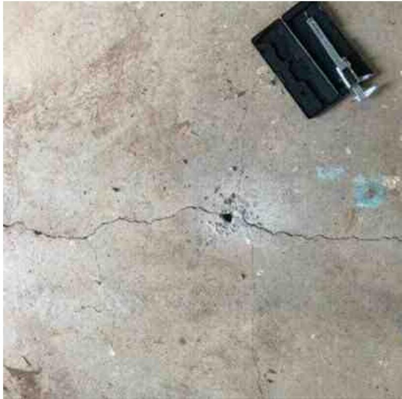
**Image 6** Drill hole in floor approximately 25mm diameter - Vernier calliper set to 25mm
