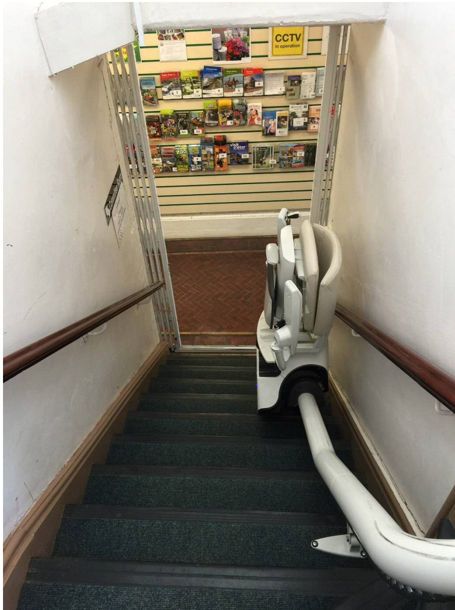
Photograph 1 – View towards Foot of Stairs, Stair Lift at Rest (seat raised)
