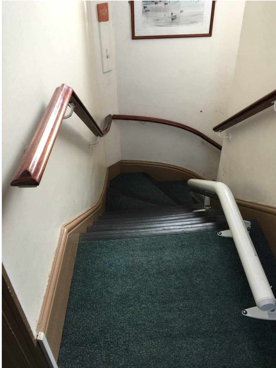
Photograph 2 – View from Top Landing towards the Tapered Treads
